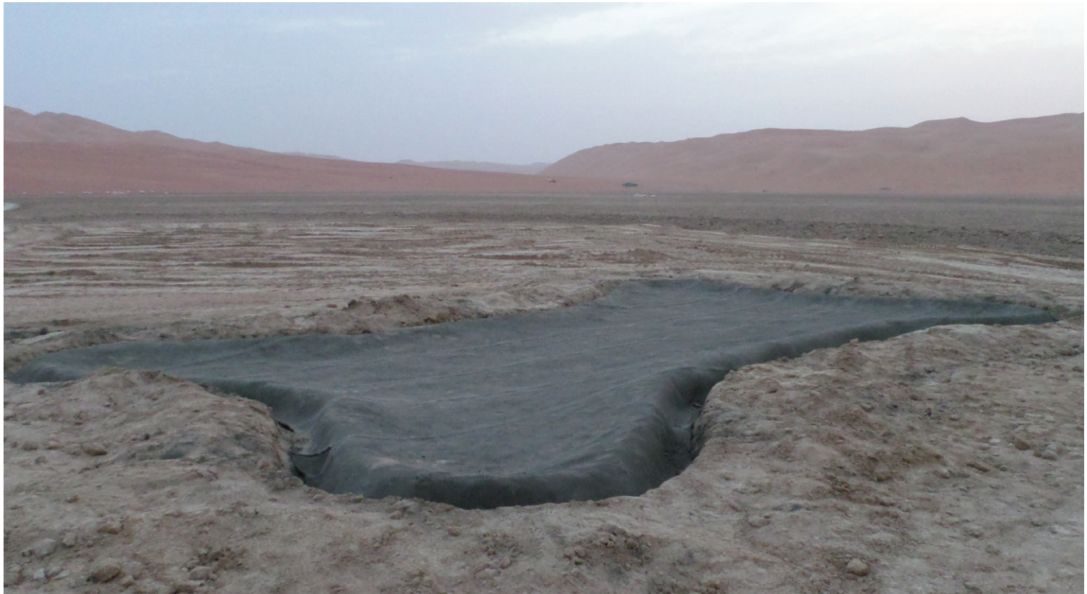
Completed pond installation
