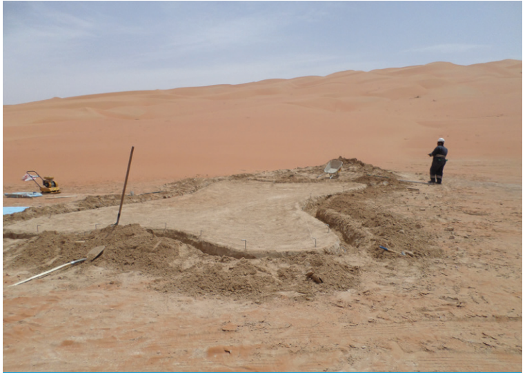
The ponds were dug with depressions in the centre for water storage
