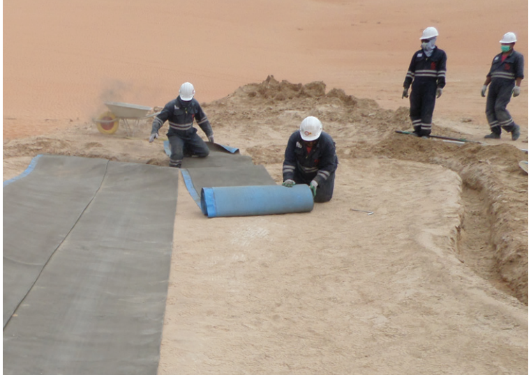
The CCH was laid longitudinally along the ponds
