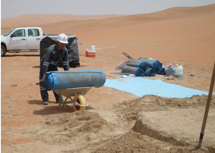
The CCH was cut to length and transported via wheelbarrow to the ponds
