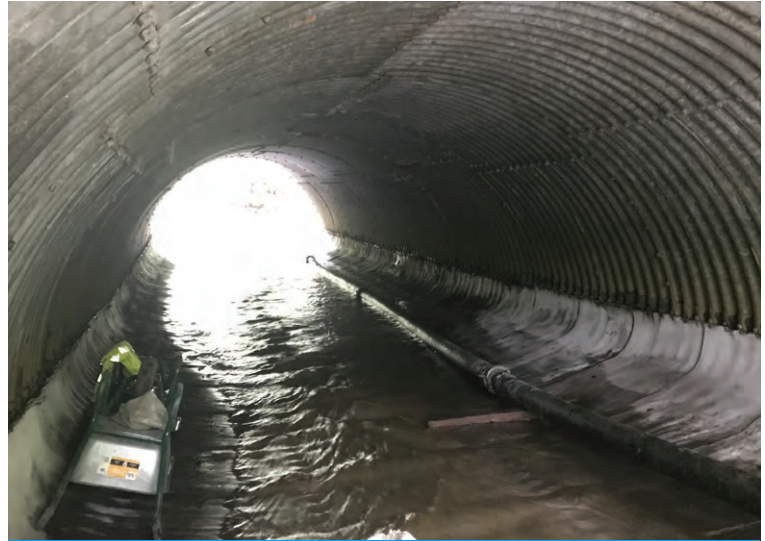
The CC was laid transversely across the culvert floor
