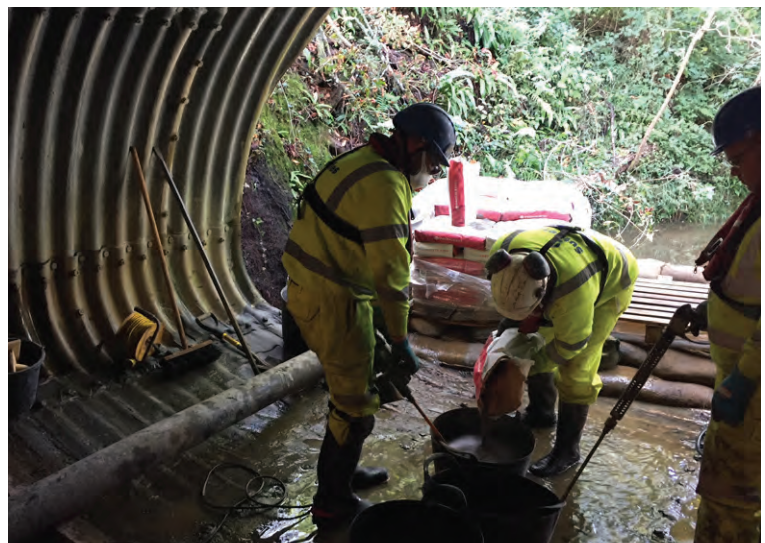
Quick-set grout was used to fill the voids in the corrugates
