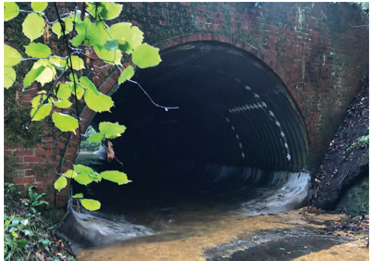
CC aprons at the start of the culvert
