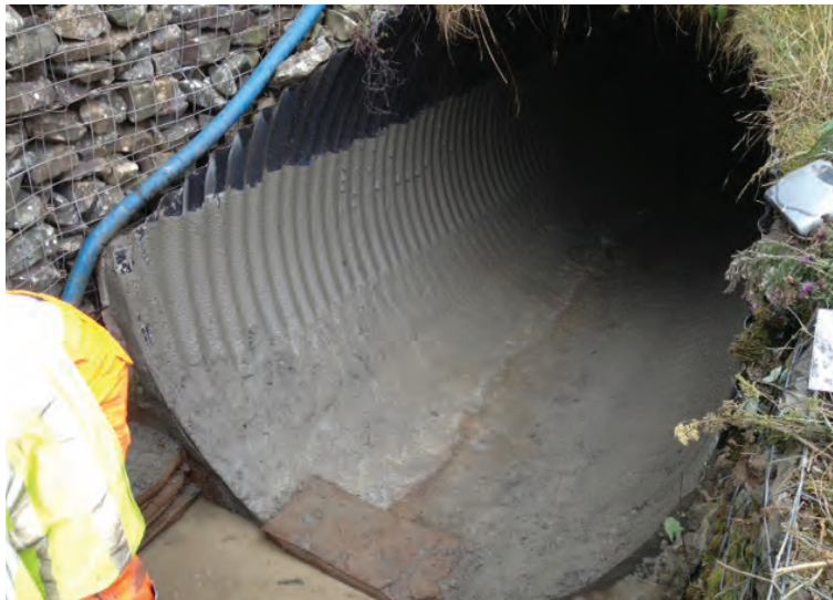
Semi-dry grout was applied to fill in the corrugations
