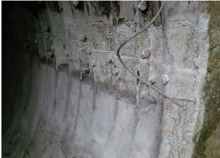
Grout applied to corrugated section
