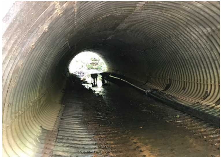
The culvert prior to prep and installation
