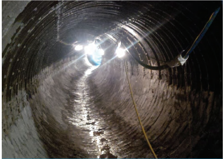
Corrugated section before works began
