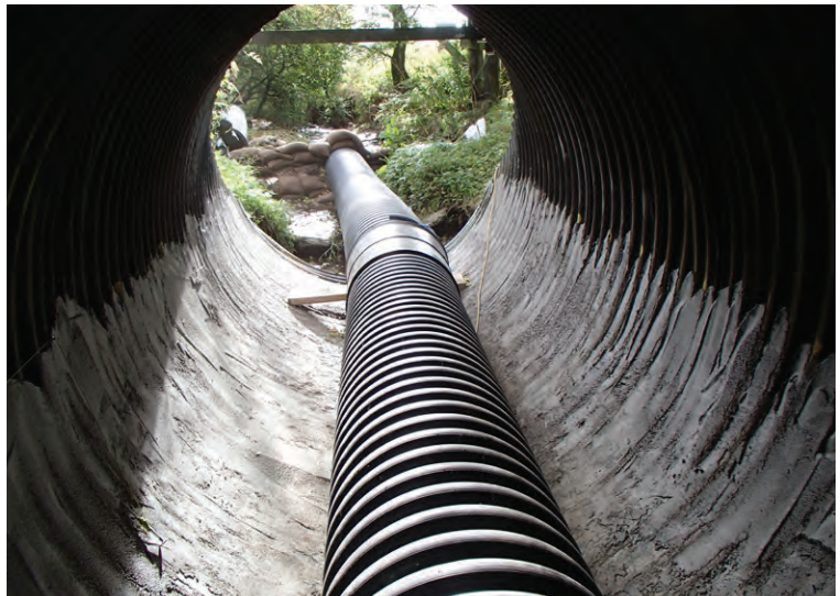
Semi-dry grout was applied to fill the corrugations
