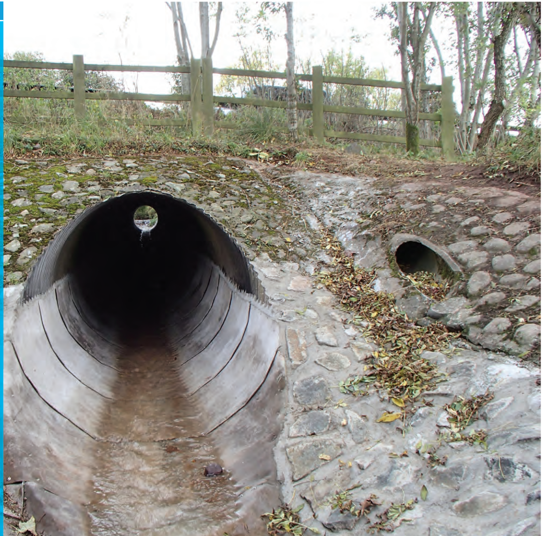
The completed culvert lining installation in Laurencekirk, Scotland.
