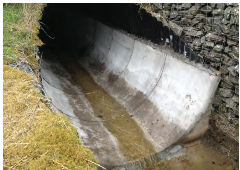
Relined culvert section
