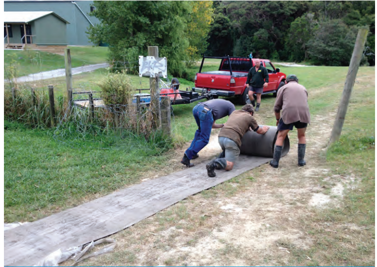
Unrolling the CC8 in order to cut it to length
