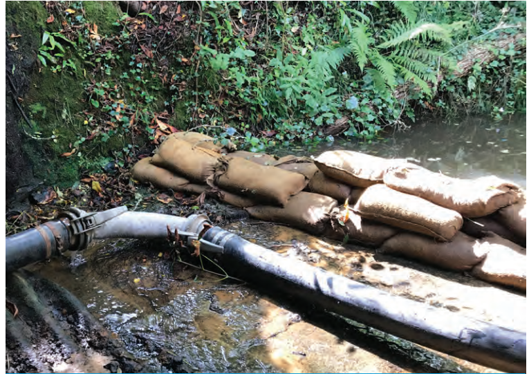
The waterflow was restricted for the works using sandbags
