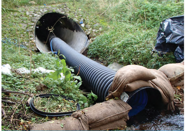
Water diverted into a 450mm HDPE Ridgidrain pipe
