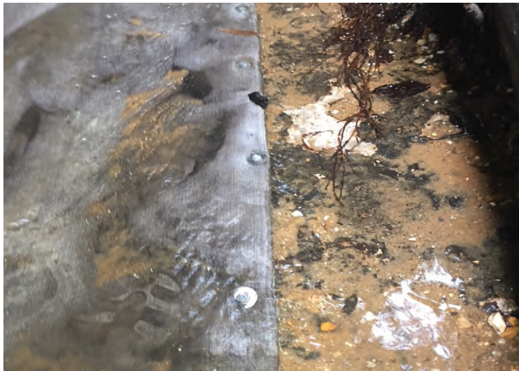
CC extending onto concrete apron, fixed using tech screws and grout
