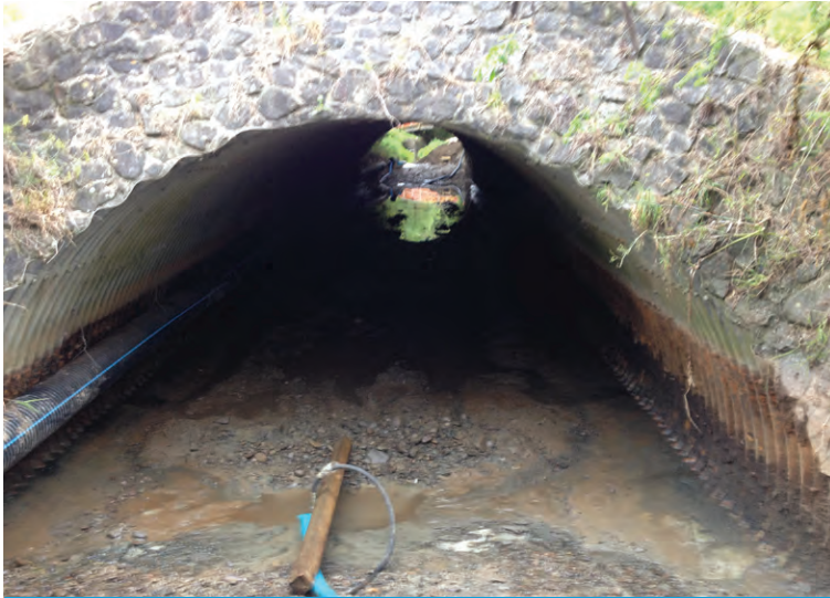
The culvert before work began
