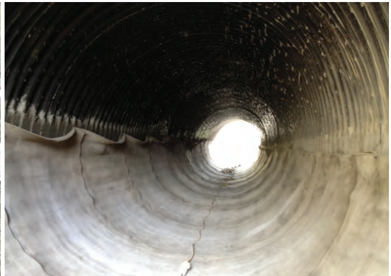
CC5 was applied in transverse layers inside the culvert
