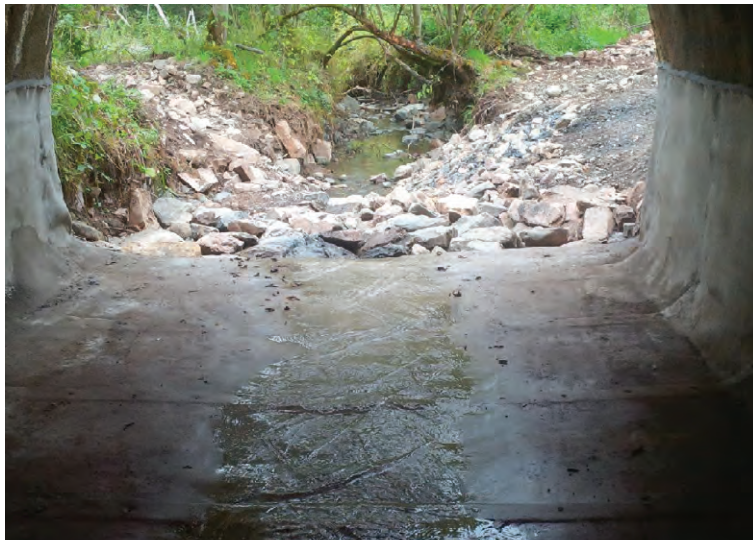
The finished install within the culvert
