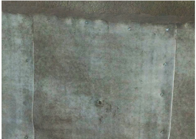
Overlaps screwed, and grout applied to prevent ingress
