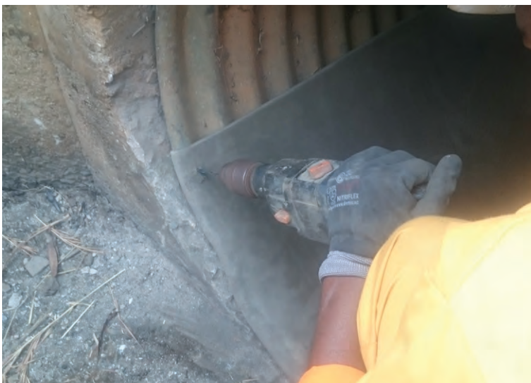
Fixing with pop rivets
