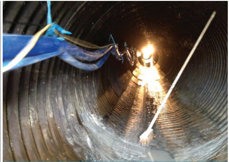
The culvert was pressure washed to remove the degraded bitumen
