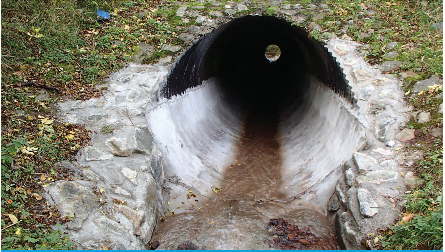
Completed relined culvert on upstream side
