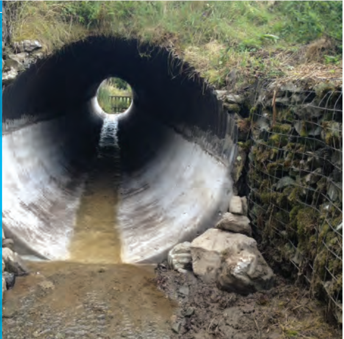
Completed relined culvert
