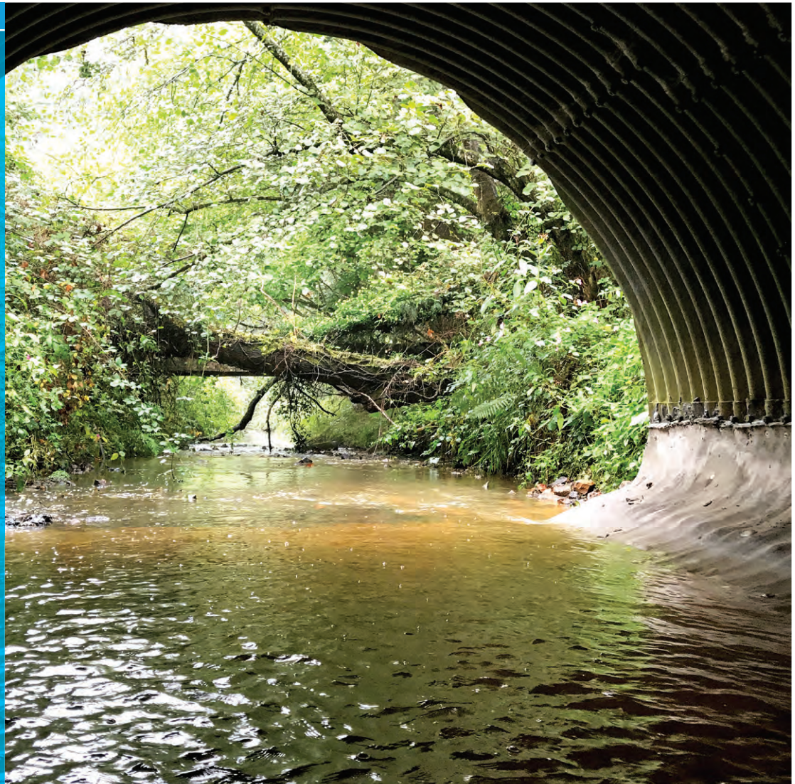
Completed culvert in use
