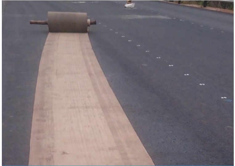
Bulk rolls were used, then cut to specific lengths on site
