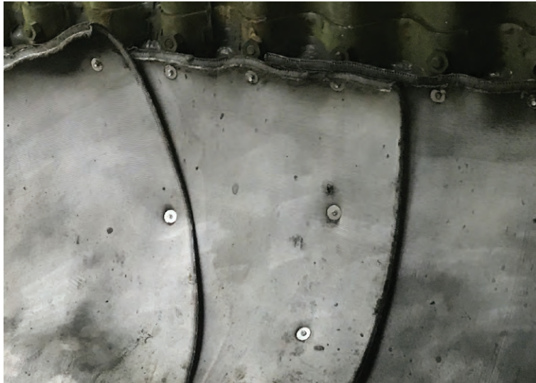
CC was fixed to the culvert using tech screws
