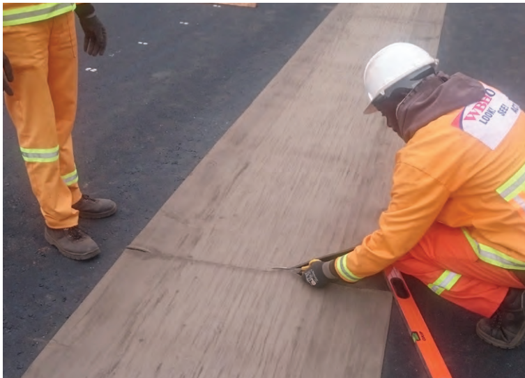
CC5™ was cut to 8m lengths for easy transportation on site
