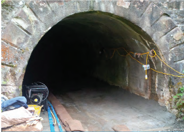
Masonry section before works began
