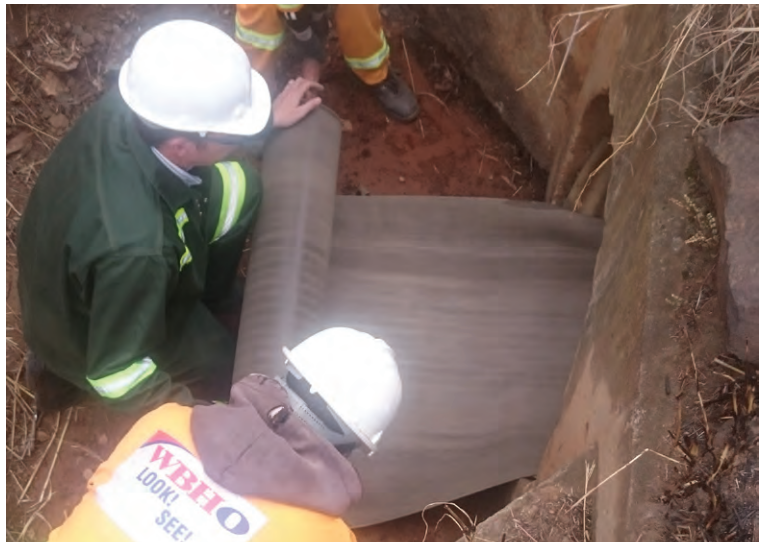
Laying CC5™ lengths in culvert
