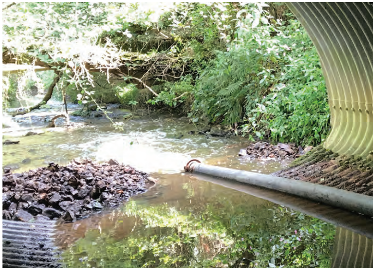
Water redirected using overpumping
