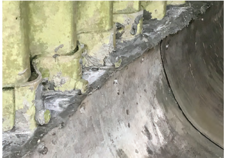
Voids behind the fixed CC were filled using more grout
