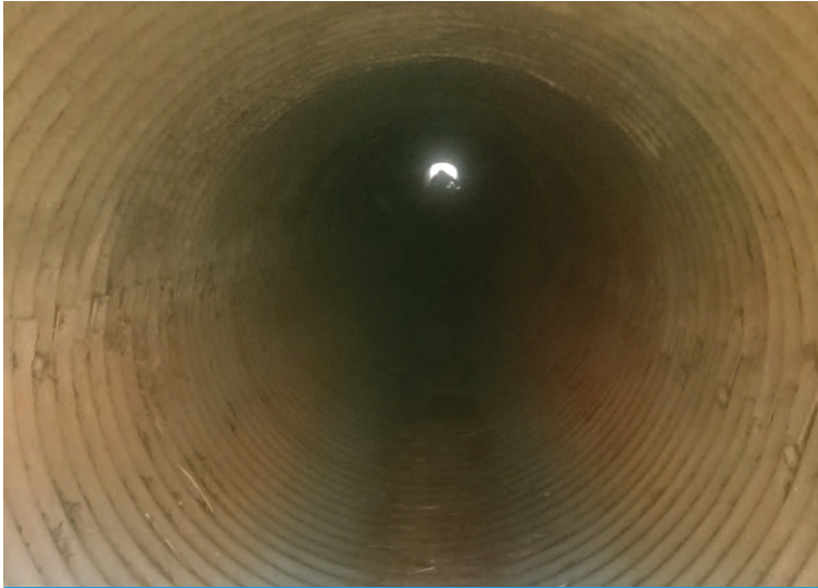
Existing corrugated steel culvert
