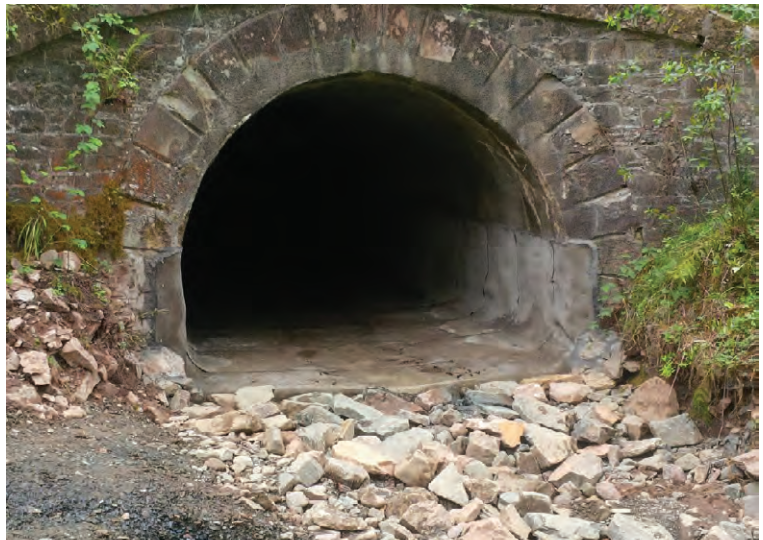
A view of the finished install from outside the culvert
