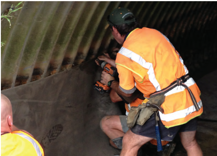
Fixing the CC to the culvert
