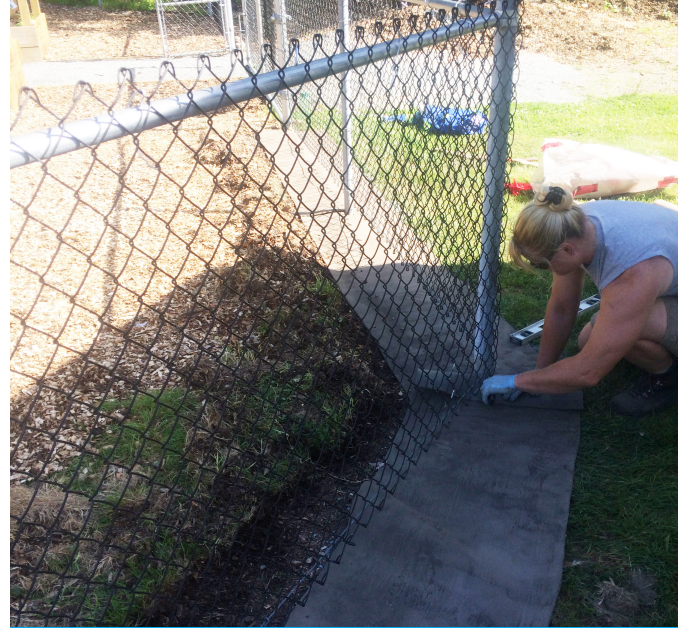
Installation of Concrete Canvas
