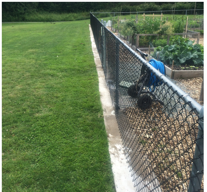
Length of completed project
