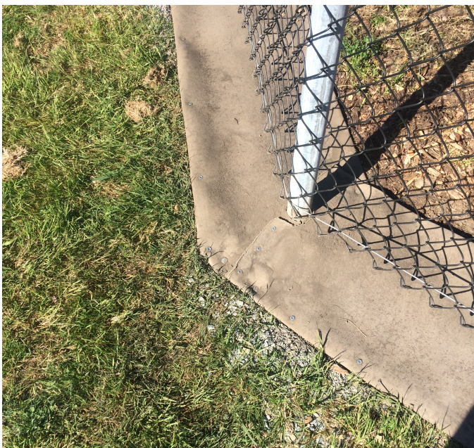
Grout used to prevent weed growth
