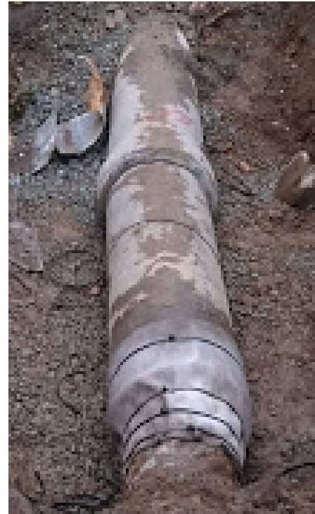
Completed CC pipe wrap
