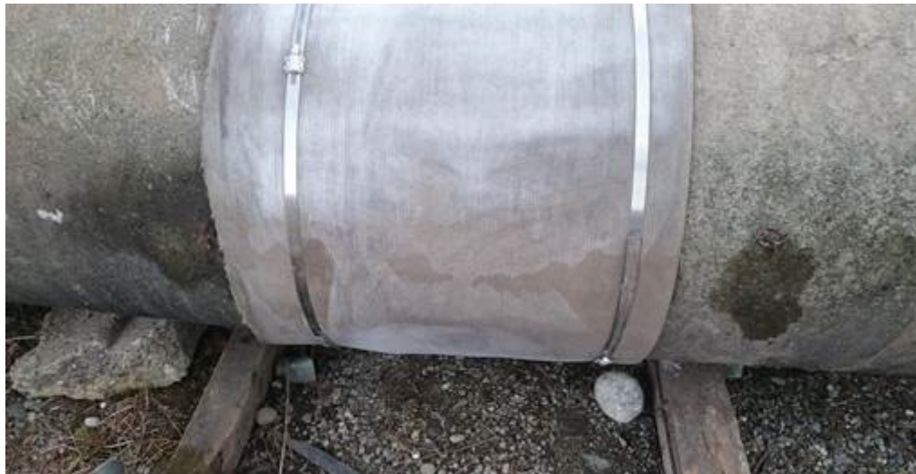
CC hydrated and set with decisions made on final installation techniques
