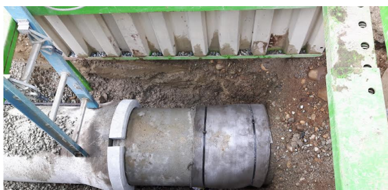
CC hydrated and set in place
