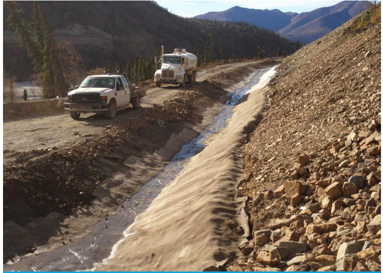
A section of the completed ditch
