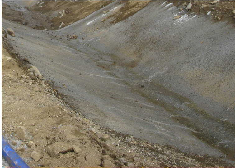
Existing shotcrete ditch
