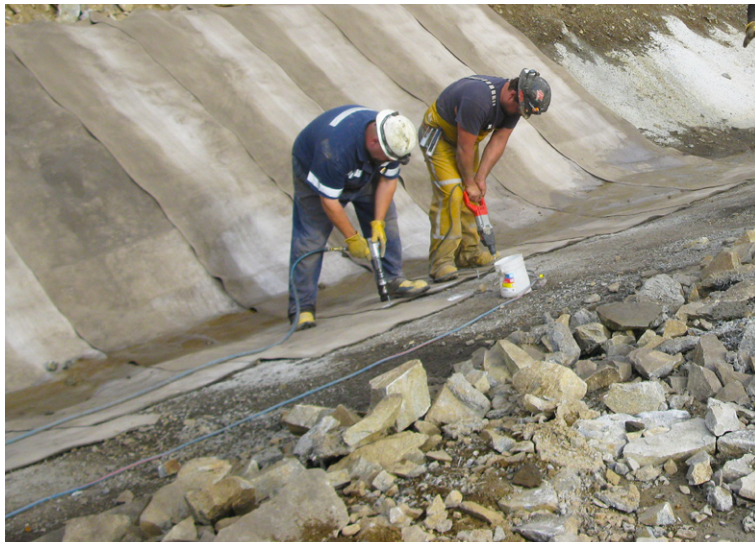
Fixing the CC to the existing concrete
