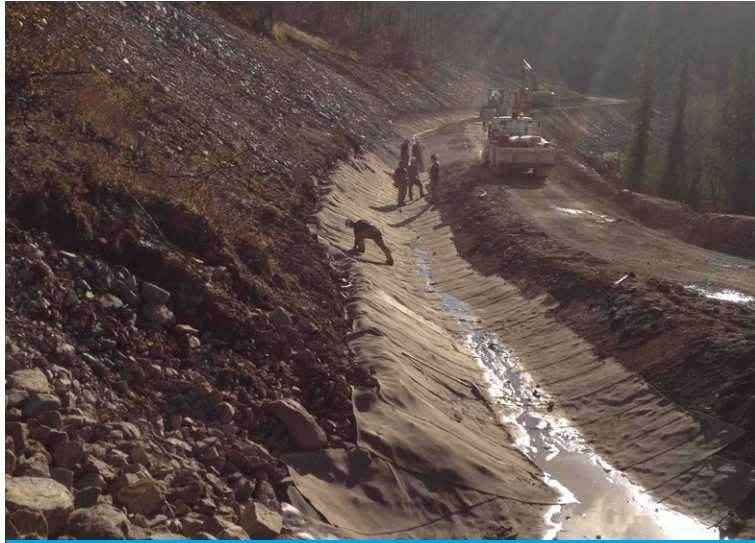
A section of the completed ditch
