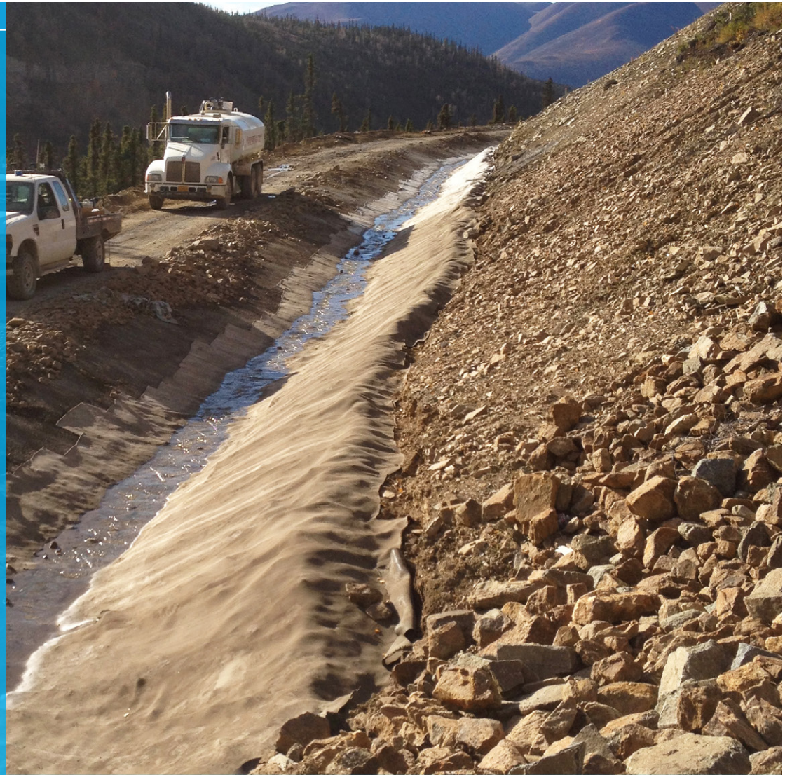
Completed section of ditch
