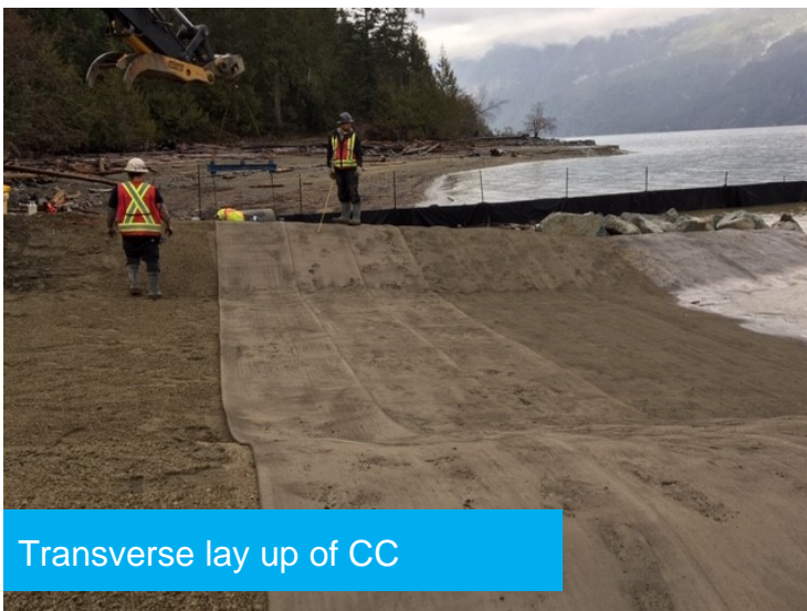
Spreader beam used to dispense bulk rolls
