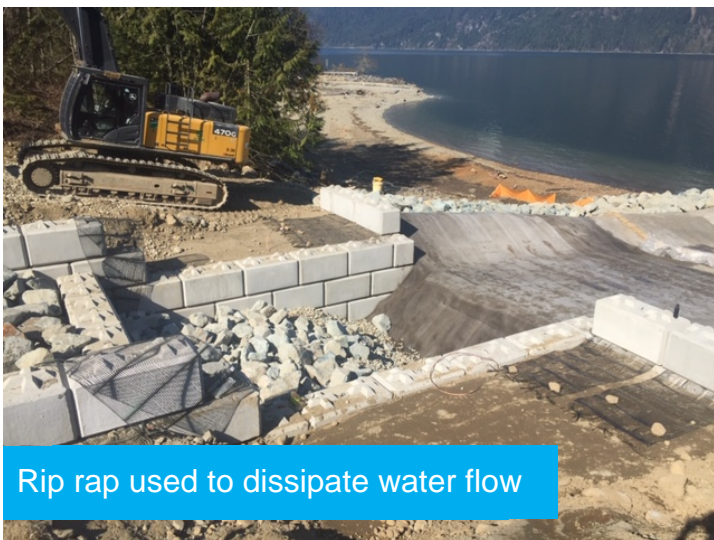
Hydration of CC after installation
