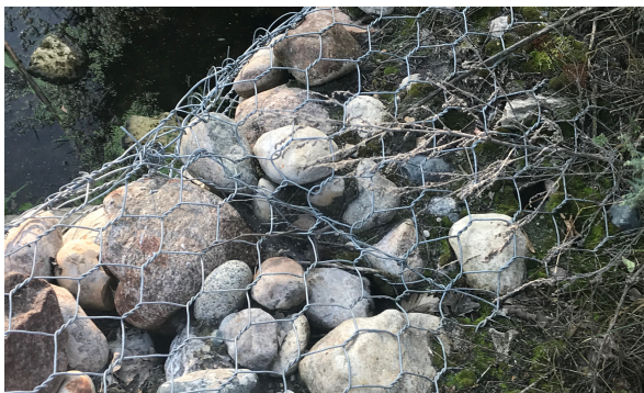
Galvanized gabion baskets with twisted wire to reinforce the shape and strengthen the rock in place.
