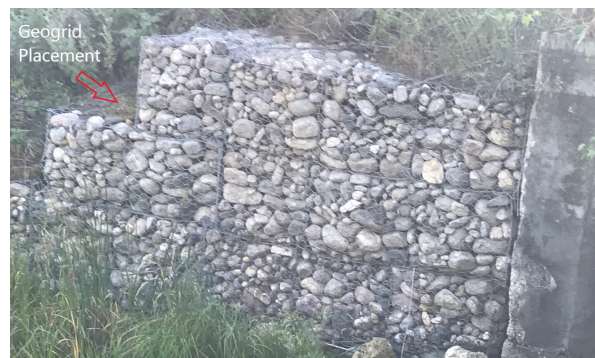
Galvanized gabion baskets with twisted wire used to hold and stabilize the wall, with geogrid placement between.
