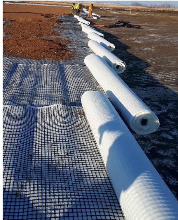
Swamp Grid™ being deployed with proper overlap.
