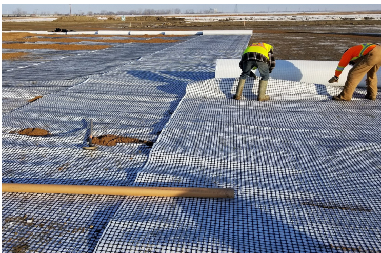
Swamp Grid™ being deployed with no wrinkles.
